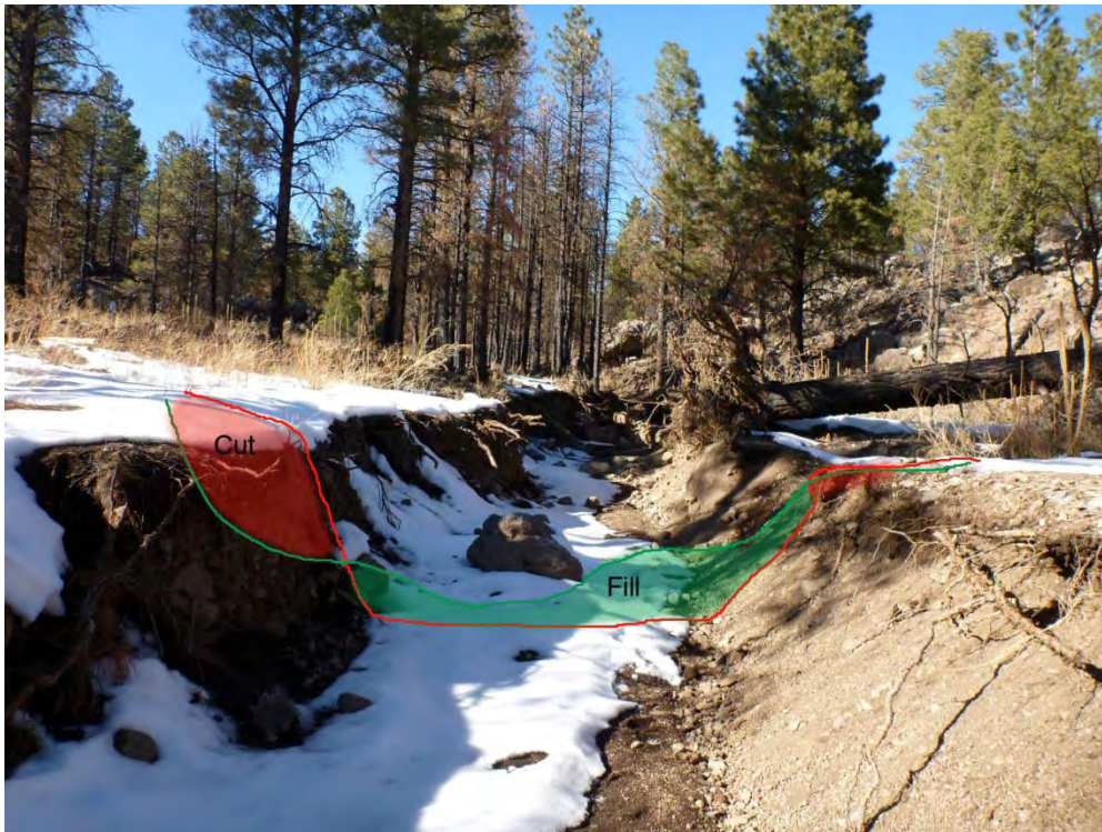
Figure 16. Typical incised channel to stable channel conversion.
