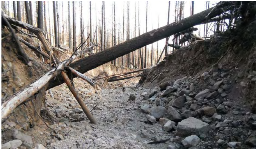
Figure 39. Photograph (ID145) of the deeply scoured portion of Peaceful Way taken in the upper portion where the steeper slopes flatten
