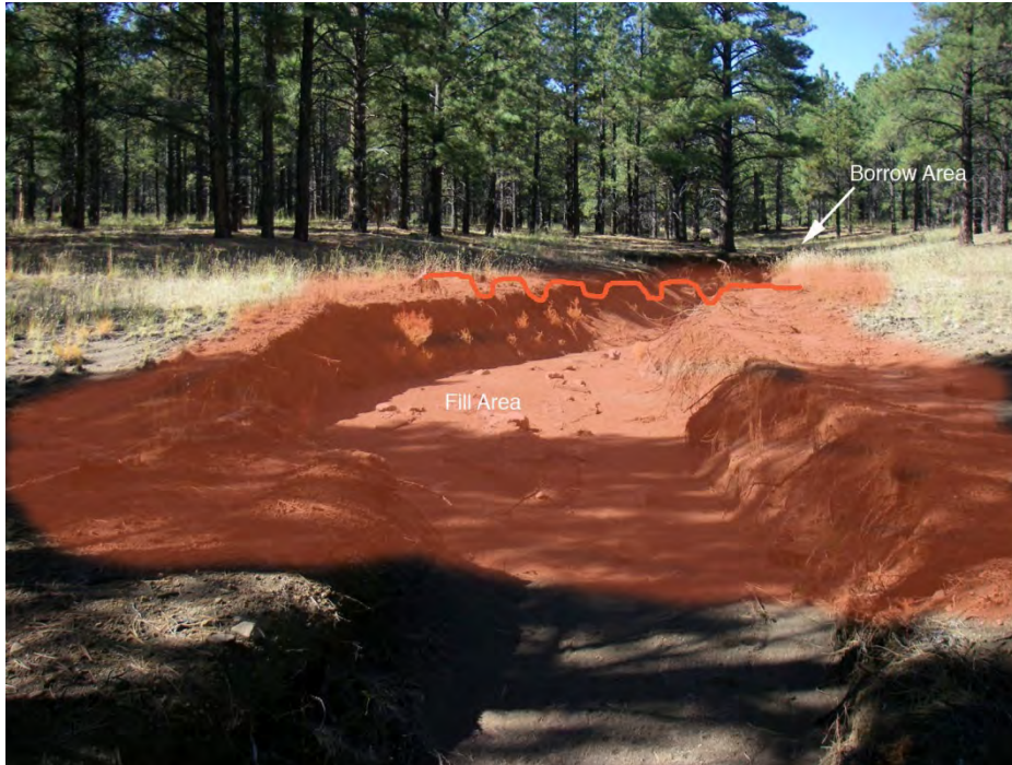
Figure 12. Typical area of fill for construction of over-widened "D" channel.
