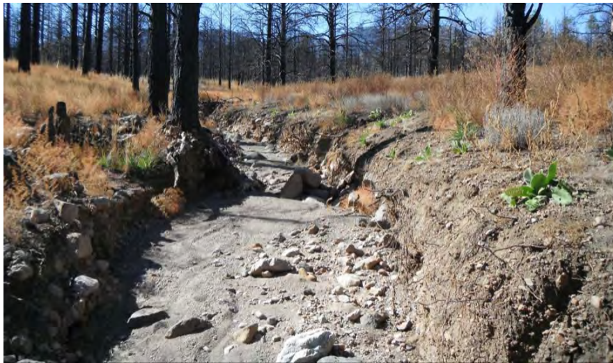
Figure 59. Representative photo (ID105) of the incision occurring through the middle-section of the Copeland watershed
