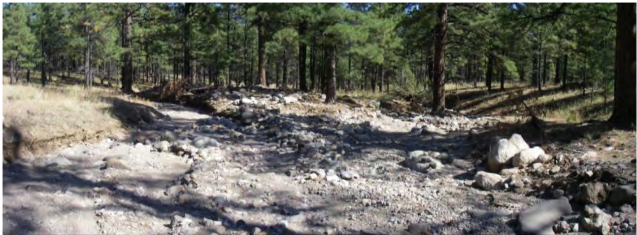
Figure 65. Photo (ID127) looking downstream showing aggradation over previously incised channel near Railroad Tank
