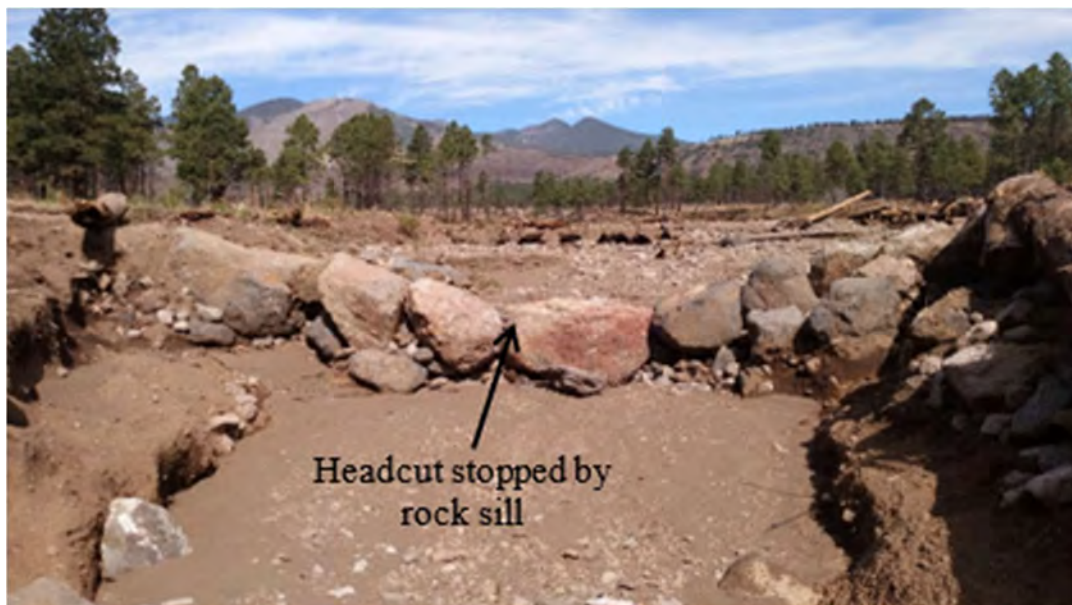
Figure 17. Rock sill maintaining upstream fan gradient in Shultz Burn area.
