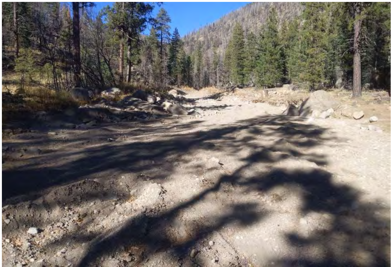
Figure 60. North tributary bulldozed cross section looking upstream.
