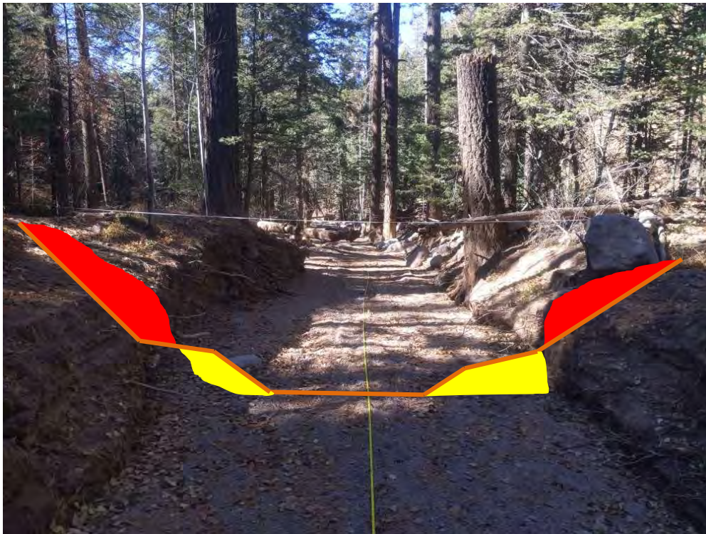
Figure 25. Typical incised channel to stable channel conversion.
