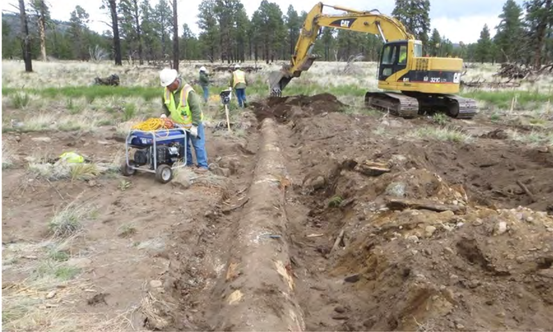
Figure 18. Log sill installation on fan surface in Schultz Burn area.
