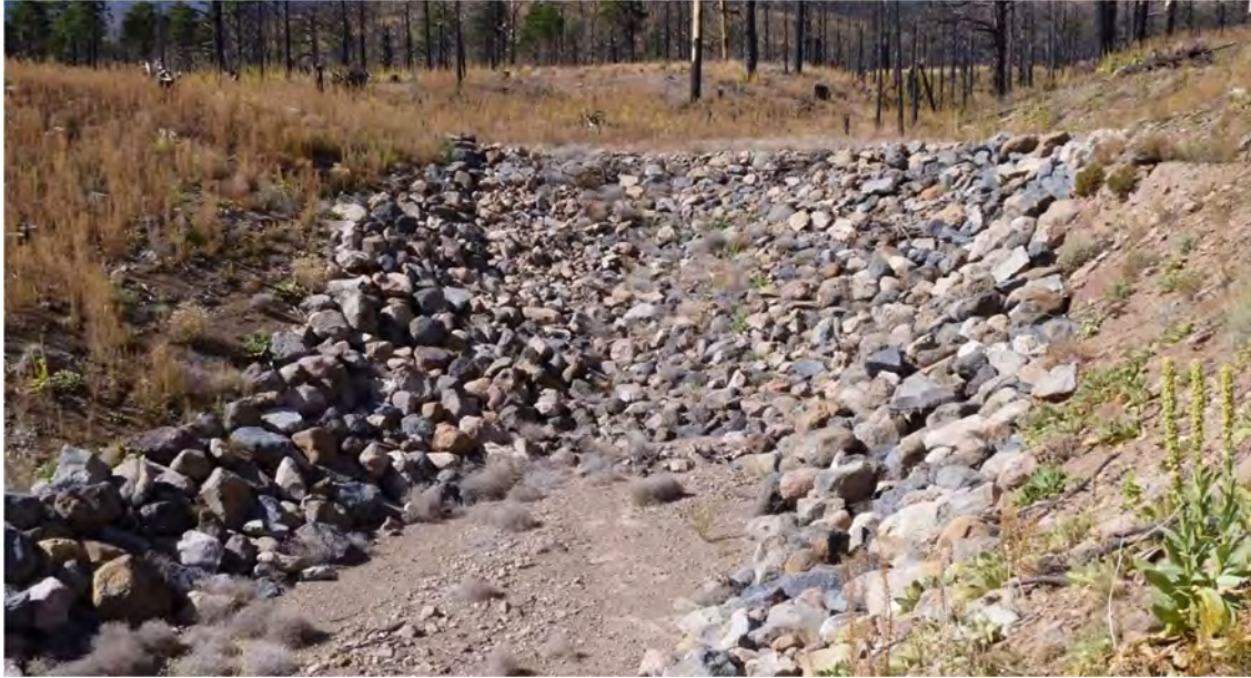
Figure 20. Rock chute in a channel at grade break caused by Schultz Pass Rd.
