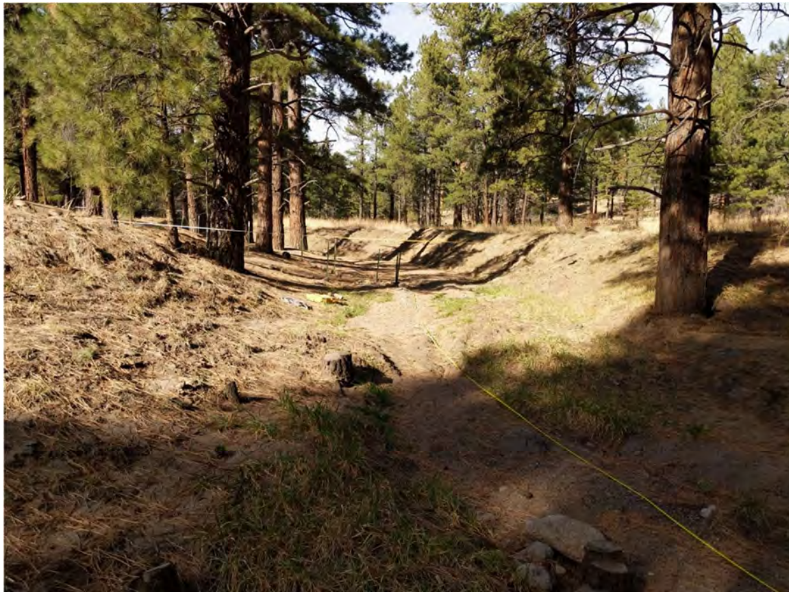
Figure 18. Spruce XS7 looking upstream.
