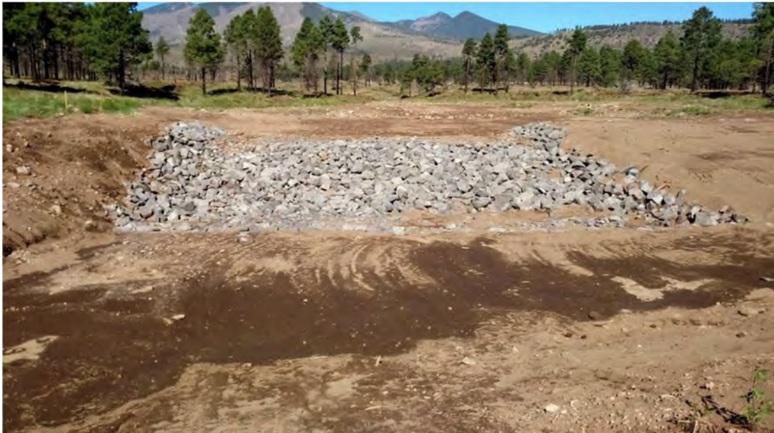
Figure 19. Rock chute at terminal trench in Schultz Burn area.
