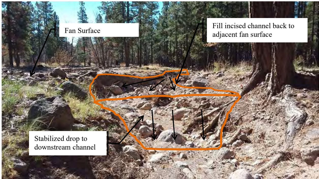
Figure 14. Typical area of fill for construction of over-widened "D" channel.
