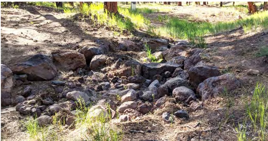
Figure 21. Cross vane weir installed in Spruce Wash channel looking upstream at weir.
