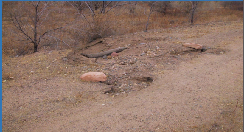
A water bar built in the low point of the road can stabilize drainage and keep fine sediment out of the gully bottoms
